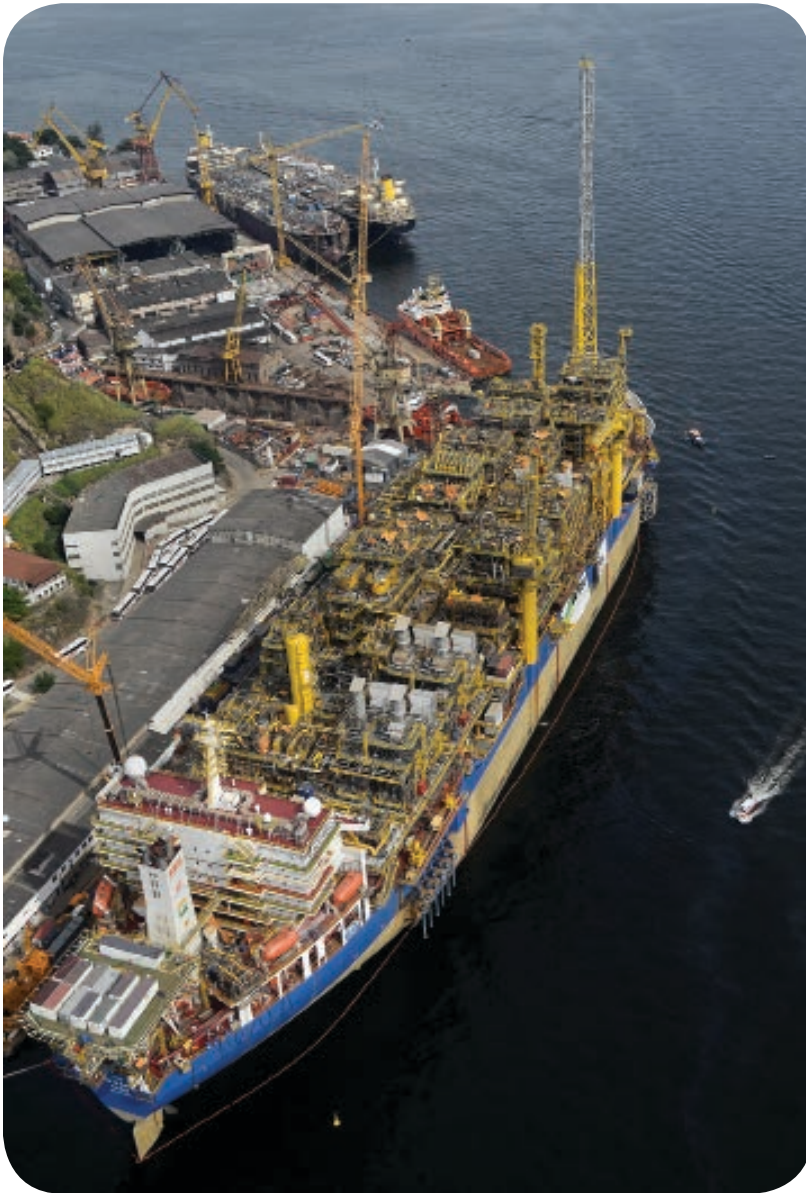
The FPSO Cidade de Ilhabela is in the final stages of construction at the SBM Offshore/Synergy joint venture Brasa shipyard in Niteroi.
